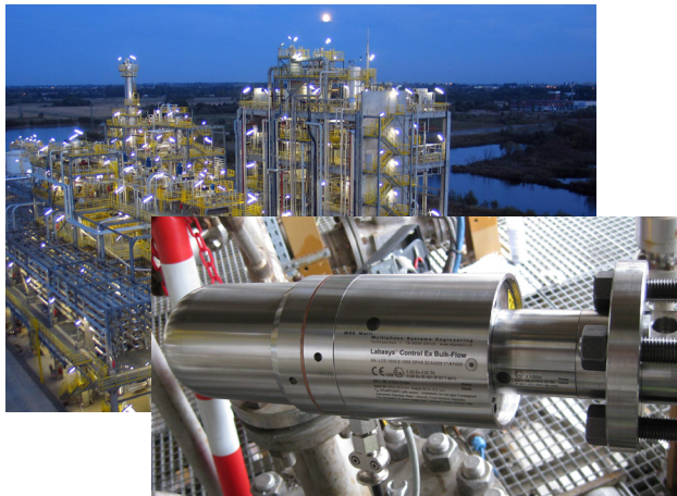
Fig. 3: Spherizone plant (left) and Labasys® Control Ex Bulk-Flow instrument at the LyondellBasell R&D center in Ferrara (right).
